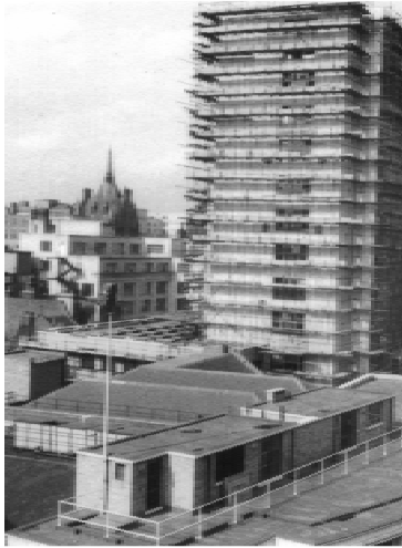
The Daily Mirror building under construction, 1960
